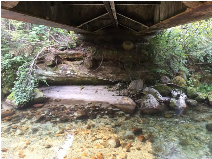
Right Bank Abutment when facing downstream
