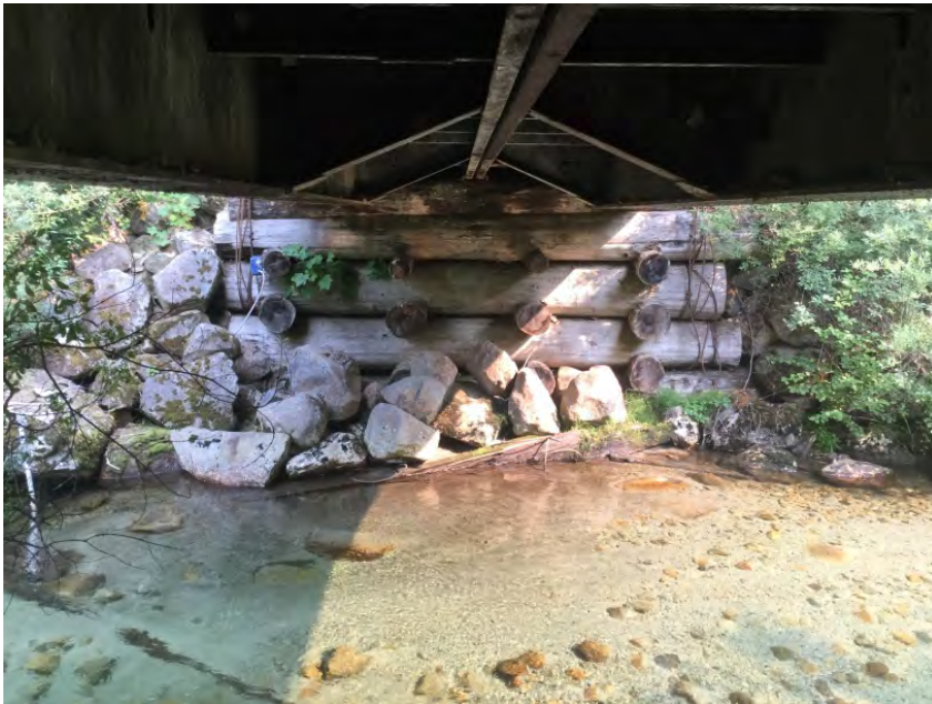
Left Bank Abutment when facing downstream
