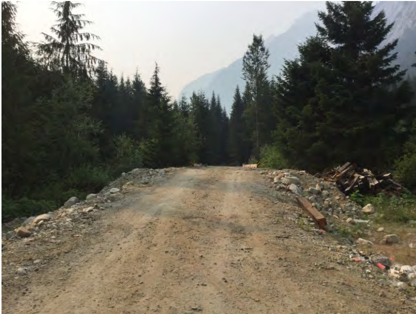
Approach from Left Bank when facing downstream
